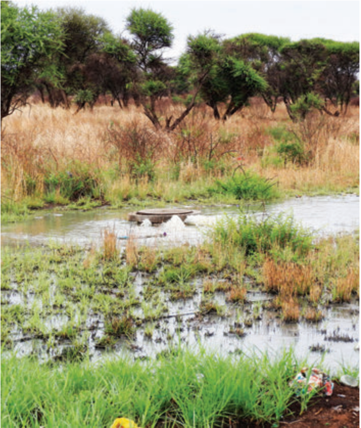
Sewerage started spilling over after a slash pump broke at the sewage plant.
